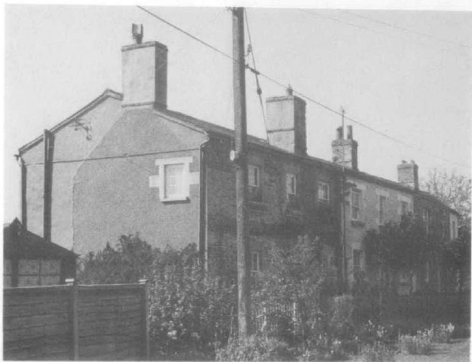
A. Ormond Terrace, Grove, from the north, showing the rebuild at the gable end and the c. 1900 re-working of the frontages.
