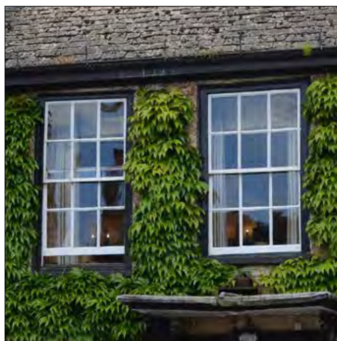
Fig. 2 Traditional vertical sliding sash windows
