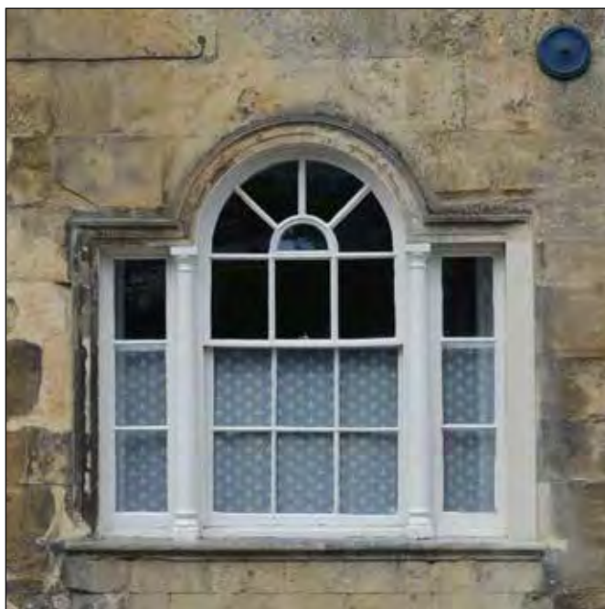
Fig. 8 A Palladian sash window in a Listed Building
