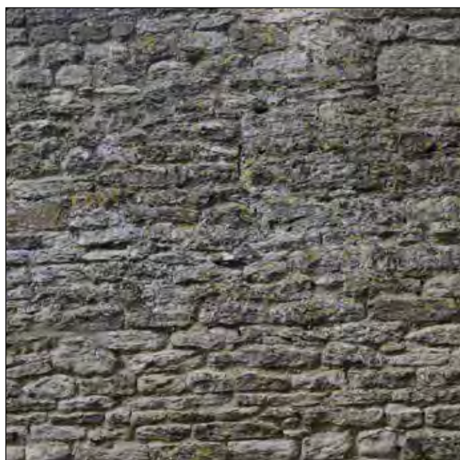
Fig. 4 Traditional rubble stone wall
