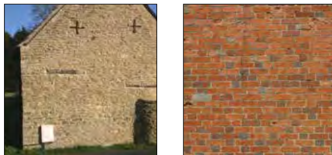
Fig. 1 Local limestone and clay brick walling
