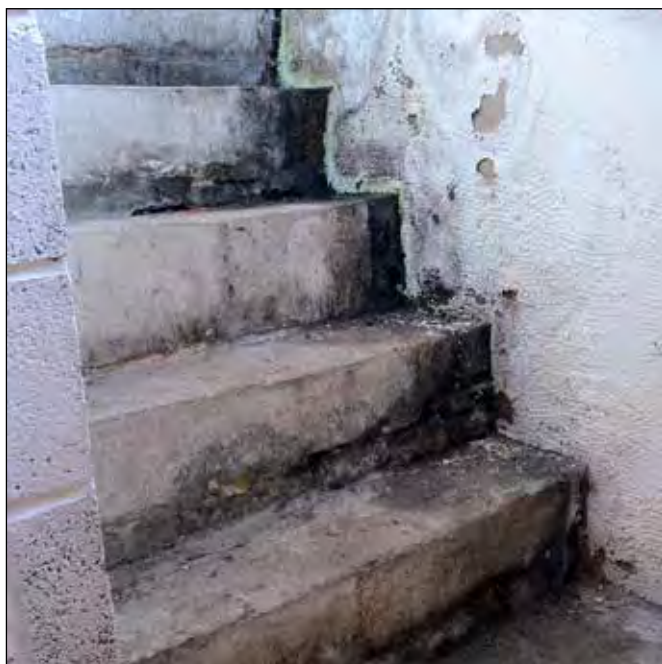
Fig. 9 Water damage to cellar steps in a Listed Building are often severe damp and condensation.
