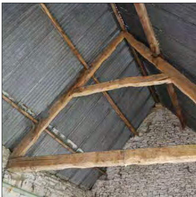
Fig. 7 Original roof trusses should be retained
