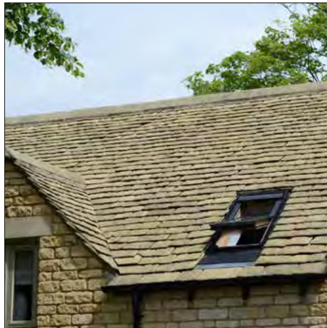
Fig. 7 Artificial stone slate roof with flush roof-light
