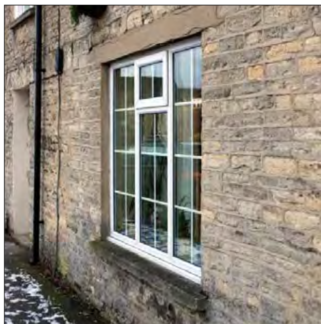
Fig. 7 An inappropriate modern uPVC double-glazed window
