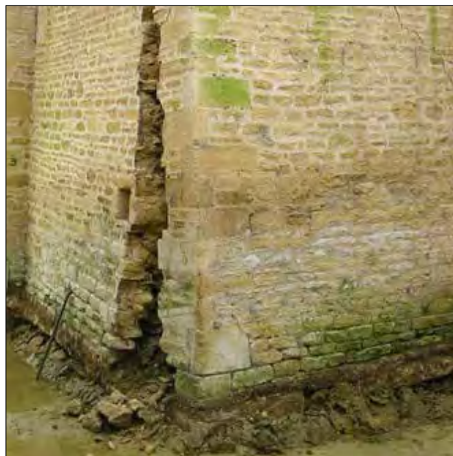
Fig. 7 Care must be taken to avoid undermining footings
