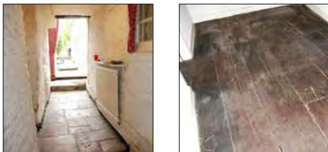
Fig. 2 Traditional stone flag flooring and elm boards
