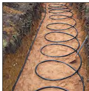
Fig. 12 Ground source pipework and air source heat pump
