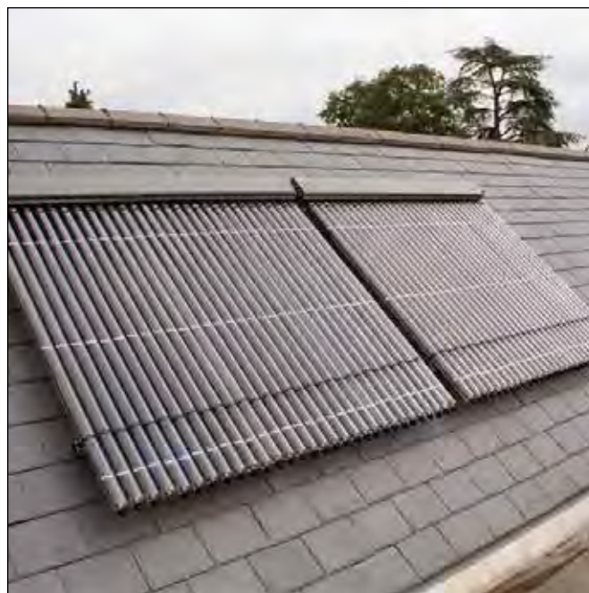
Fig. 14 Solar thermal panels (evacuated tube type)
