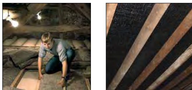
Fig. 6 Insulation can be laid between joists or rafters
