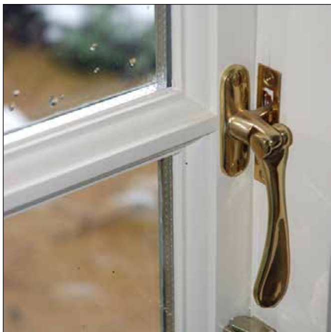
Fig. 9 Slim double-glazing with well detailed glazing bar
