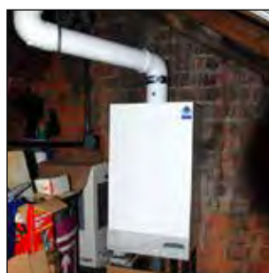
Fig. 11 Combi-condenser boiler, and flue next to chimney
