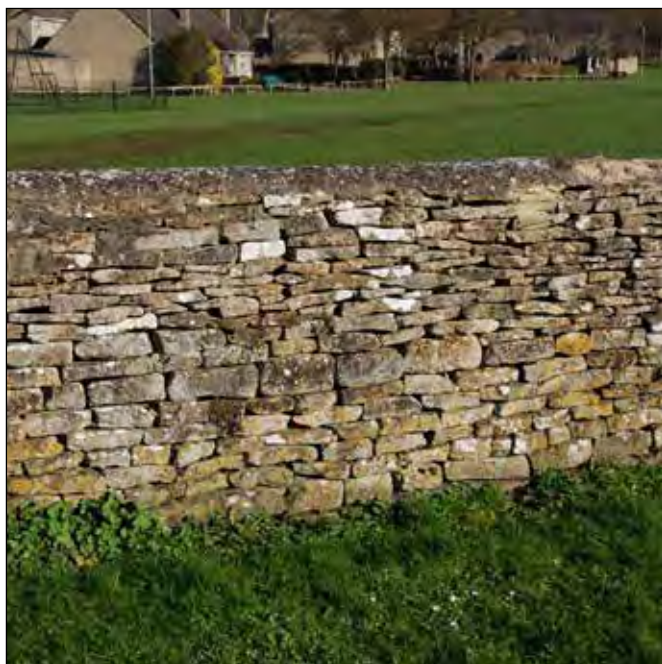
Fig. 1 Traditional dry stone wall
