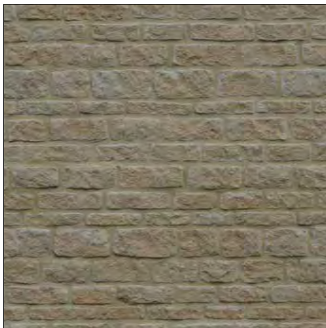
Fig. 8 Artificial stone wall
